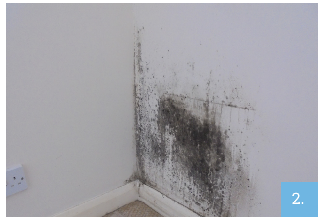
Condensation mould in the corner of a room exposed after furniture removed.
